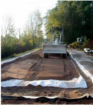
Fig. 2 An example of product re-use in road building [3].
