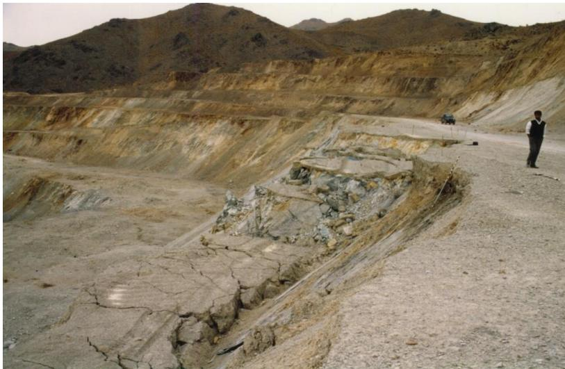
*Figure 7 : South west slope of Sar Cheshmeh copper mine in Iran. Overall view and wedge failure mechanism*
