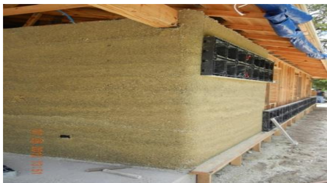
Figure 2. A hemp-based house built in Florida (with permission from Bob Clayton, Florida, USA) [103].
