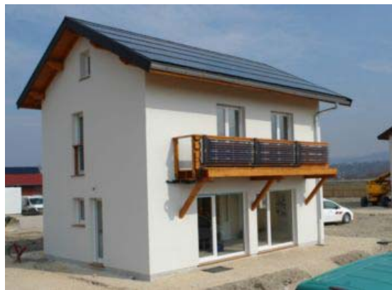
Figure 4: view of the house (west and south façades)
