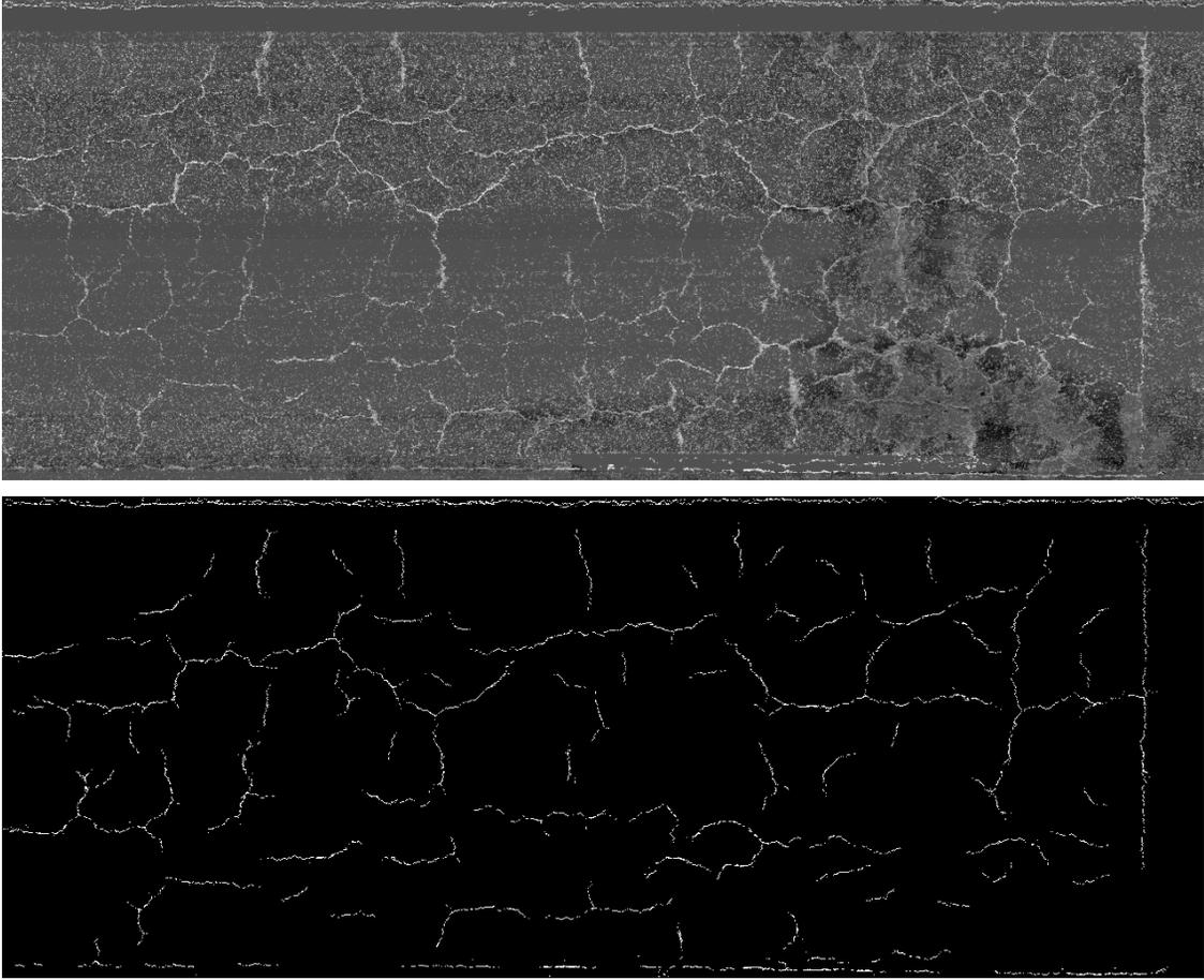
**Fig. 7.** Detection of road cracks. (top) original, 11294x4096 image, (bottom) the cracks obtained for  $L \geq 100$ ,  $k = 65$  and  $r = 0.15$ . The sliding window is a  $100 \times 100$  rectangle.
